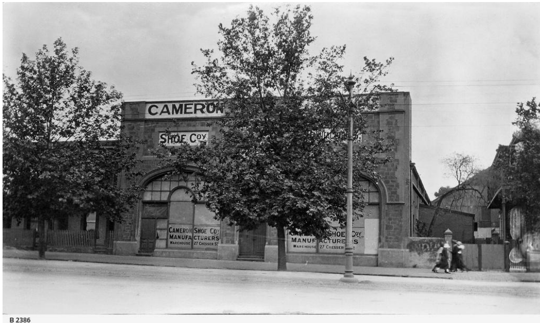
State Library of South Australia - Cameron Shoe Company [B 2386, Cameron Shoe Company premises on North Terrace; left side is 121 yards east of Morphett Street. Frontage is 21 yards. Demolished in 1928. 1924, Photographer, State Library of South Australia. Part of Acre 10 Collection.
